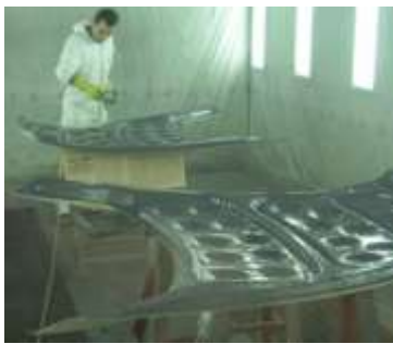
Figure 16a. Primer coat being applied to the completed hood assemblies.
